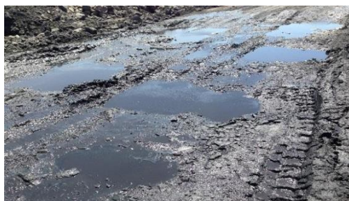
(a) Potholes formed on the haul road
