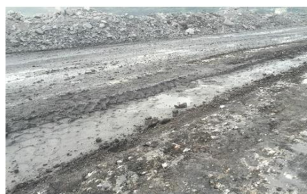
(a) Potholes formed on the haul road
