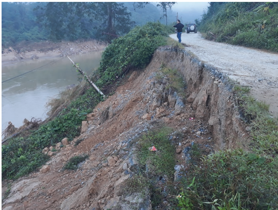
Fig. 6.8 Flash floods damaged crop fields and electricity and transport infrastructures along provincial road in the Van Chan district (Source: An Thinh Nguyen 2017)
