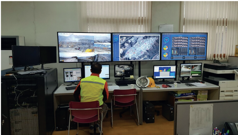
FIG. 3 Example of an ICT-based mine safety management system corresponding to smart mining digital twin <Level 2> [1].
