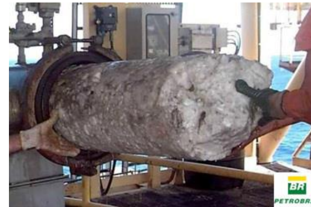
(Hydrate recovered at slug catcher-Petrobras)
