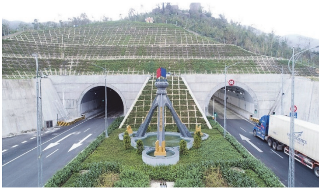
Figure 1 The DeoCa tunnel
