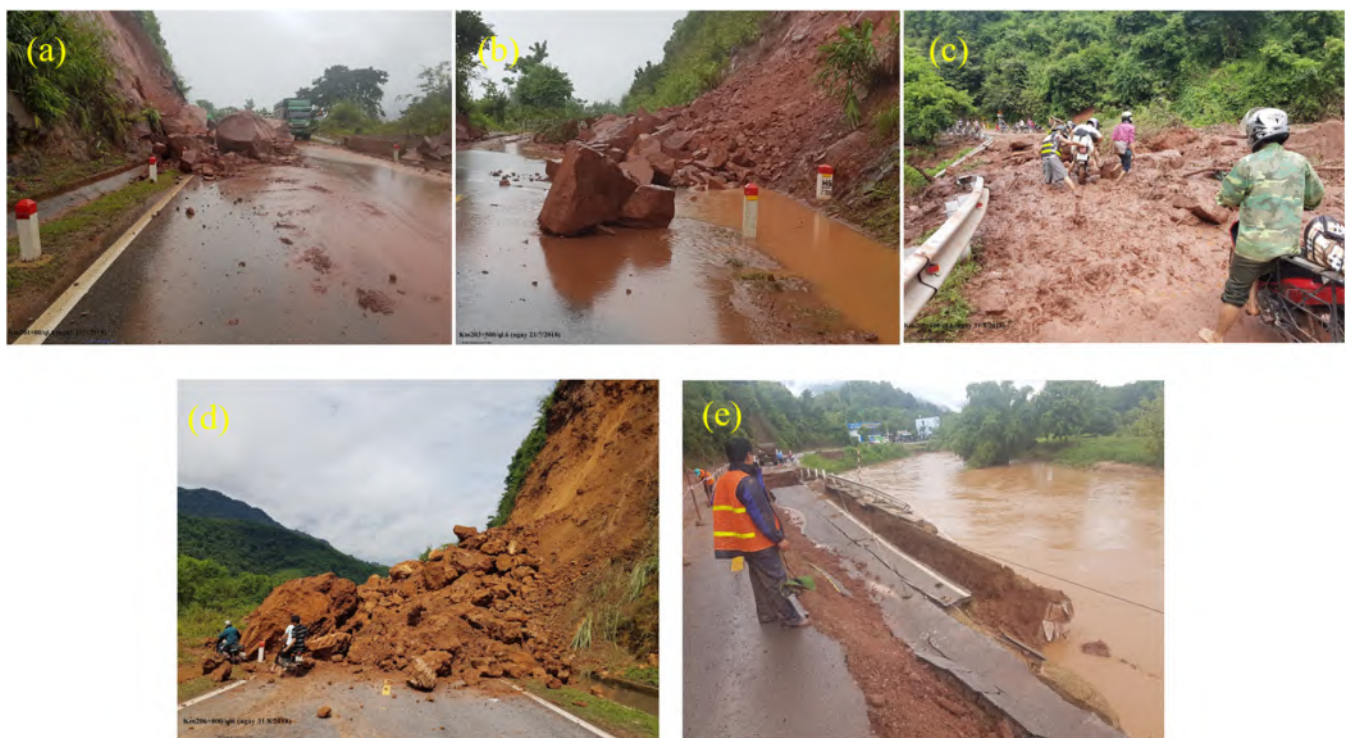
Figure 2. Some images of landslide events on Highway 6 in the Son La province in July and August 2018 through field surveys: (a) At Km 201 + 00; (b) At Km 203 + 500; (c) At Km 205 + 100; (d) At Km 206 + 800; and (e) At Km 230 + 300 (provided by Road Joint Stock Company 226, located in Son La province, Vietnam).
