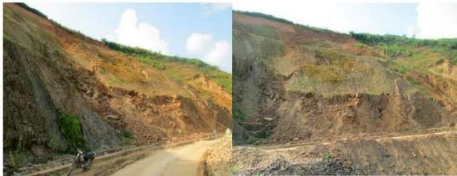
Figure 2. Two photos of the landslide on the slope wall of National Road 279, near the right bank of Nam Kim stream, Na Pa village, Muong Kim commune, Than Uyen district. Source: Vietnam Institute of Geosciences and Mineral Resources [29]
