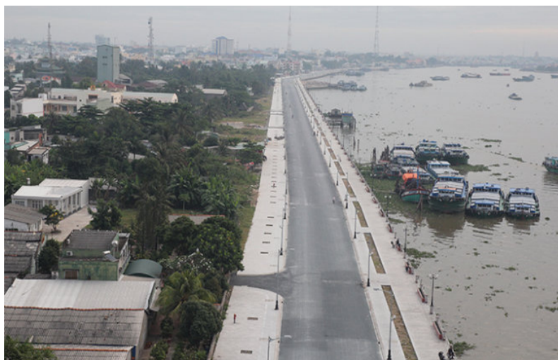
Fig.19. Road and Tien River embankment project in My Tho City, Tien Giang in 2015
