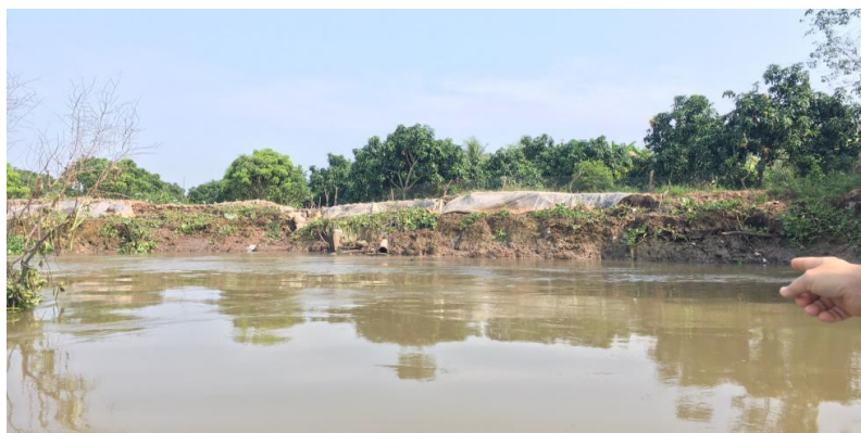
Fig. 10. The riverbank erosion in a curved river section in Cai Be District (2020)
