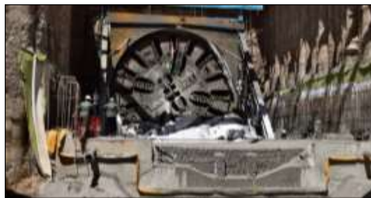
Figure 5. The cutter-head of TBM (TURL2 Project)
