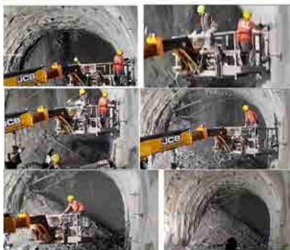
Figure 1. A Tunnel collapse process (taken from a video clip).
