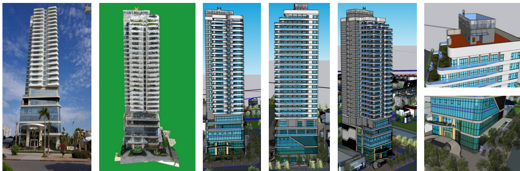
Fig. 13. The 3D LoD-3 model for a high building from point clouds UAV and TLS on Sketchup Pro 2021 software
