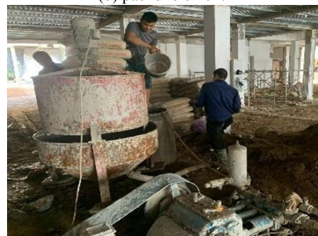
(d) grout mixing and pumping machine
