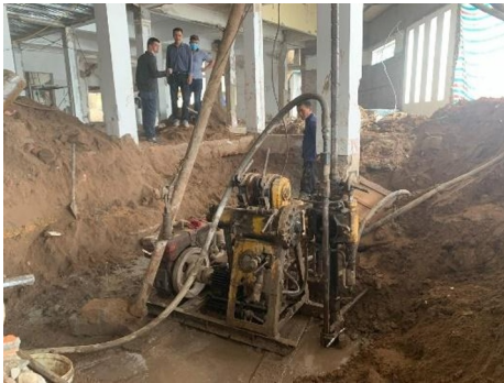
(a) drilling the grouting hole
