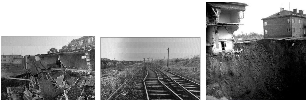
Fig. 2. (left) Garages in Karol Swierczewski Street were completely collapsed by a huge sinkhole on 5 th August 1977, (middle) railway tracks were broken in the Wapno village [25], (right) A huge hole in the Wapno village, which was allegedly caused by land subsidence triggered by mining exploration in the Tadeusz Kościuszko salt mine [26].
