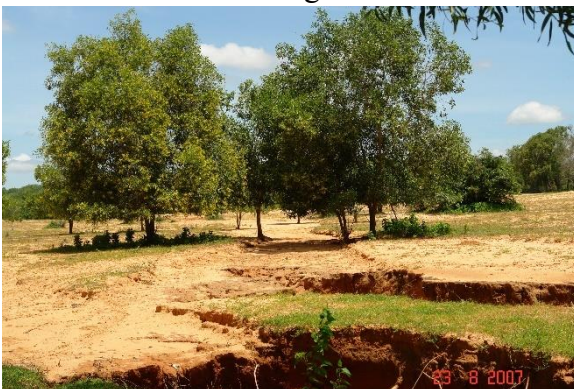
Figure 5. Drainage zone at the tip of an eroded ditch Tien Hoa village area
