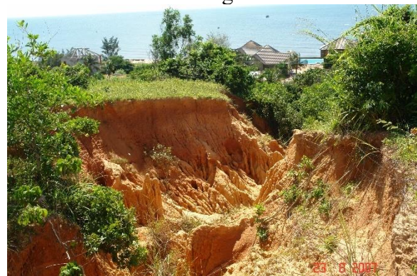
Figure 6. Developing ditches in Tien An village
