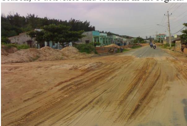
Figure 1. Sand floods cause houses and roads to be buried
