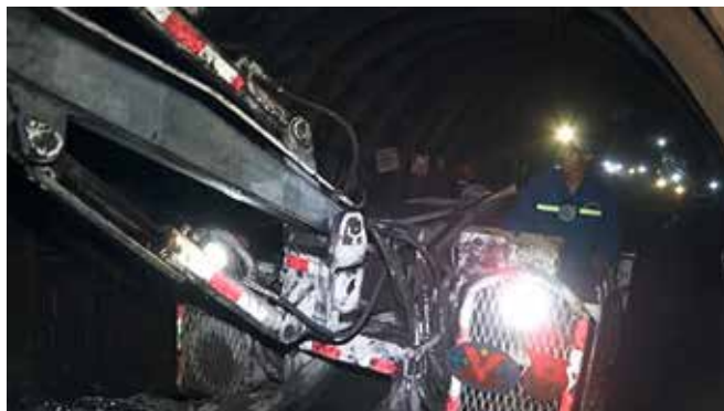
b. Excavators in the working face
