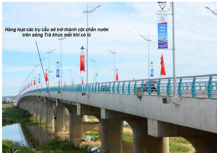
Photo 3. A series of piers are obstacles to water, reducing the ability to drain water on the Tra Khuc river
