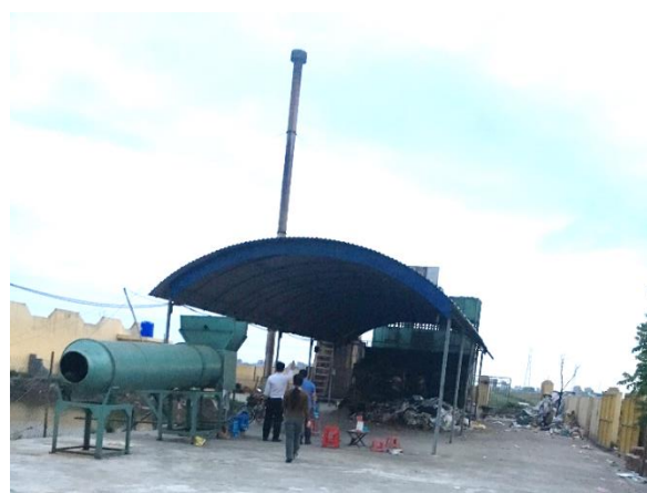
Figure 5. The incinerator with emission treatment system by absorb in the sanitary landfill in Xuan Ninh commune, Xuan Truong district.
