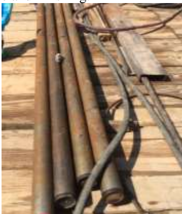
Fig.1. Jet grouting triple type rod used in HCM MRT Line 1
