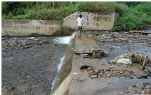
Fig. 1. Deposition blocks upstream and paralyze water collecting system of weirs in the Northwest
