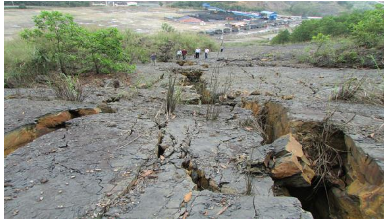
Fig. 5. Cracks in siltstone and sandstone formed by the impact of the tailings pit and the mining network near Khe Cham coal mining site in Quang Ninh.
