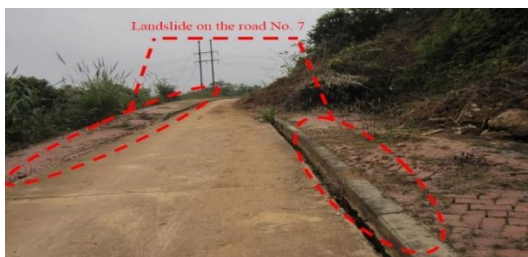
Fig. 9. Cracks on road 7 behind the substation
