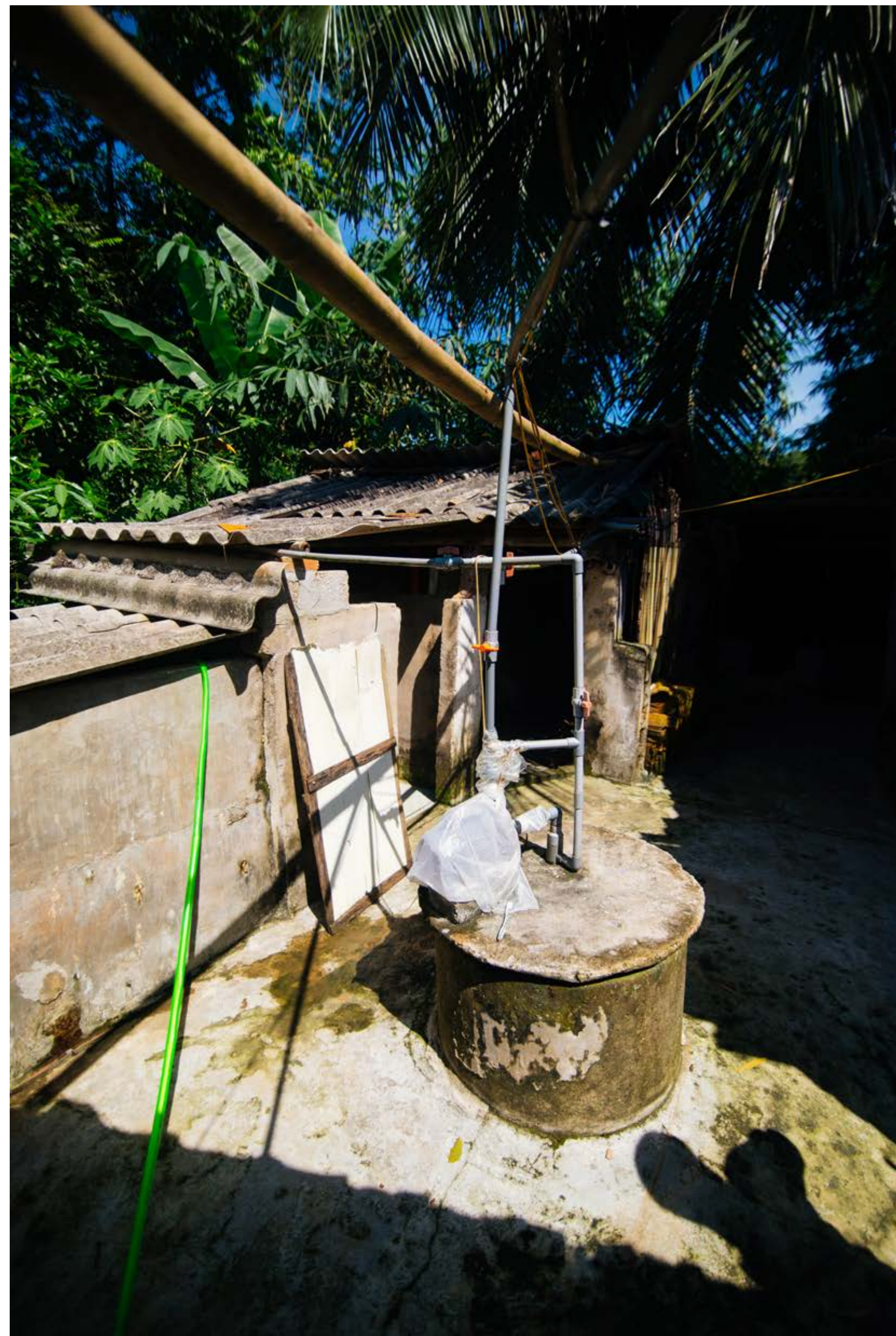
Photo: Contaminated wells and temporarily equipped water purifiers
