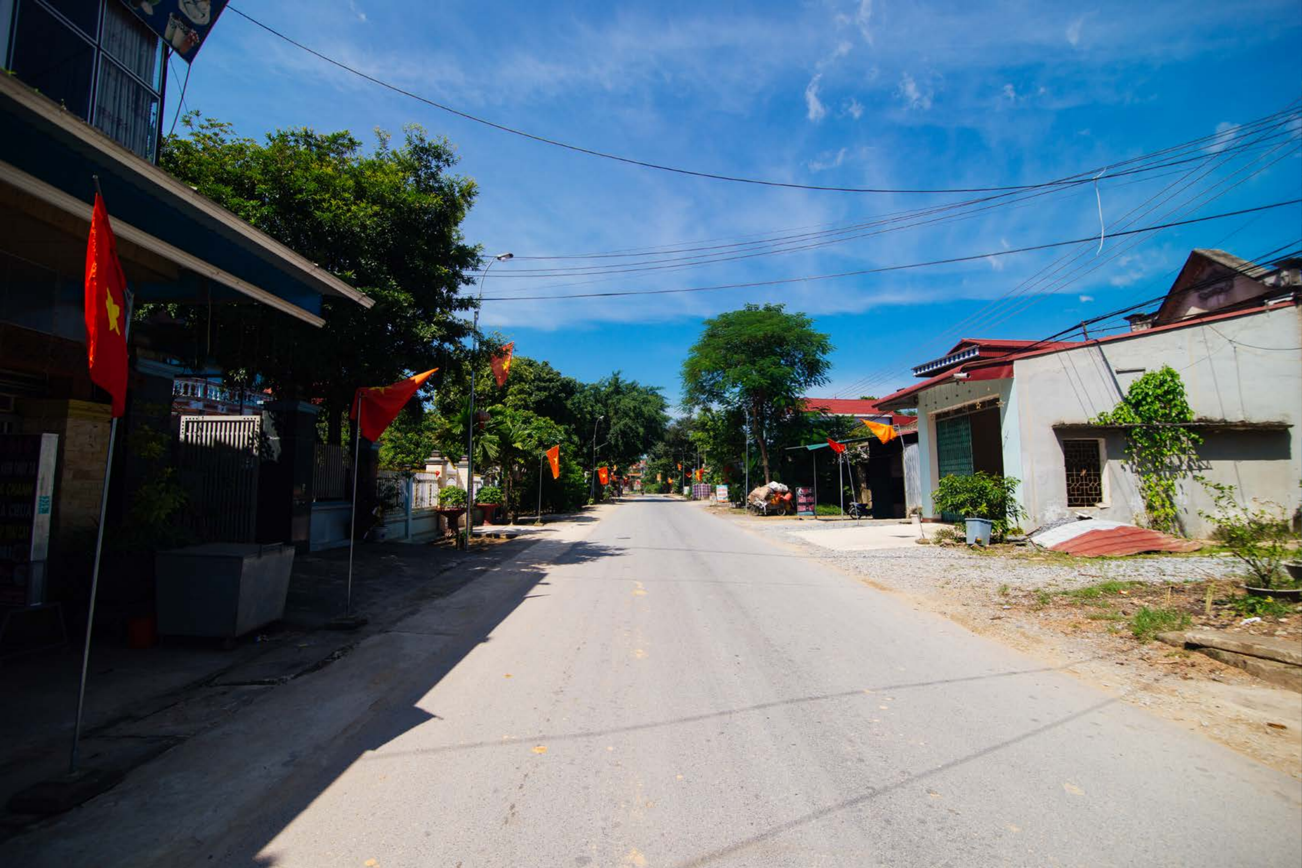
Photo: Provincial Road 217 runs through Thanh Long village
