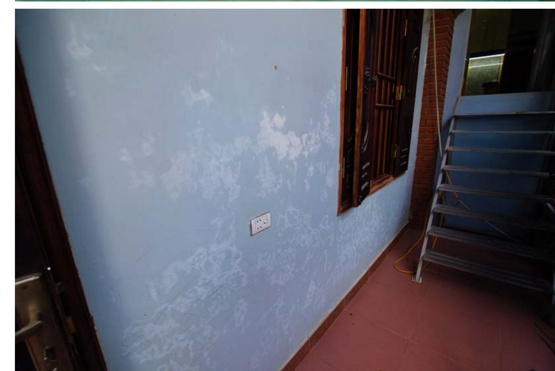
Photo: The walls with flood water stains
