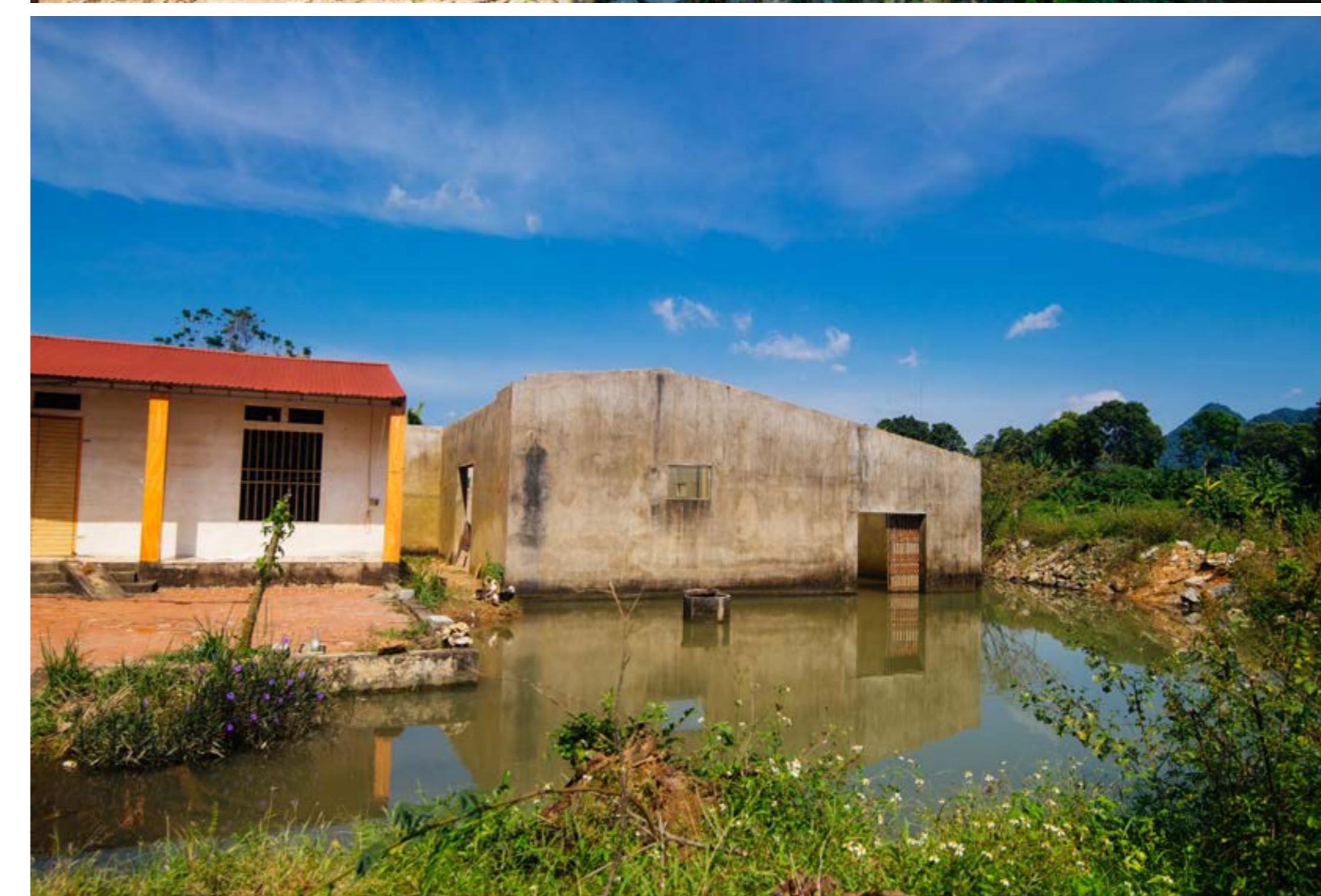
Mr Mai Xuan Duc standing in front of his mother's 4-level house, his house and factory, which are now flooded with water
