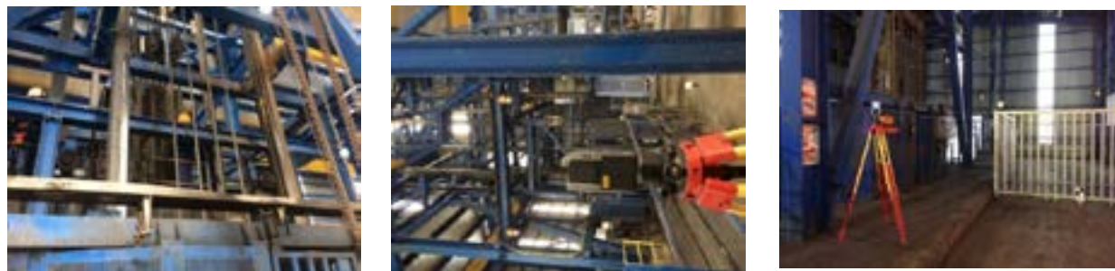
Figure 8. Columns and beams in the headframe of the mine shaft.
