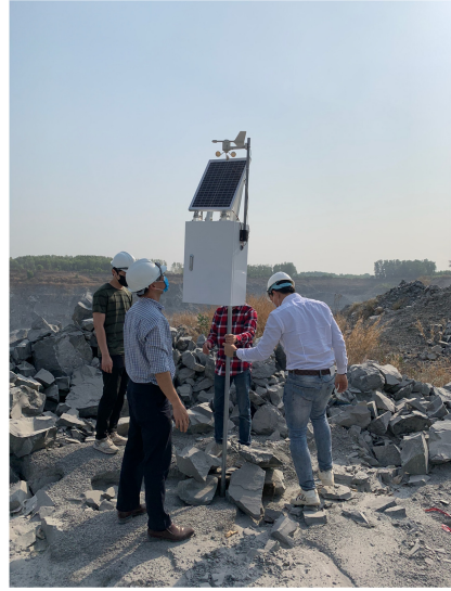
Fig. 9. Installation of the monitoring systems for temperature, humidity and wind speed at Nui Beo coal mine
