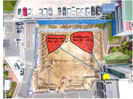
Fig. 5. Aerial view of the in-situ test site
