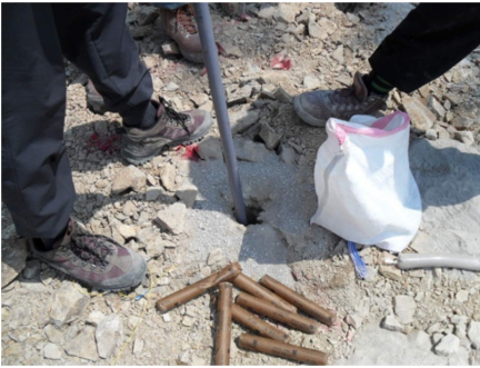
Fig. 6. Cleaning up the blast hole
