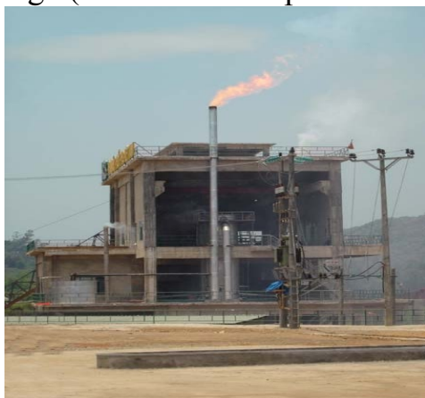
Photo 1. Producing yellow phosphor at the industrial park
