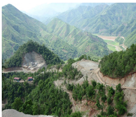
Figure 2. Ban Phuc Nickel area overview – looking to northwest explosives magazine in centre left and upper ROM pad centre right.
