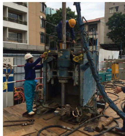
Figure 14. Jet Grouting work at Saigon Opera House
