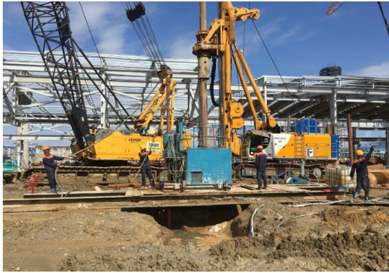
Figure 5. Jet grouting work in Hoa Phat Dung Quat Iron and Steel Complex Project
