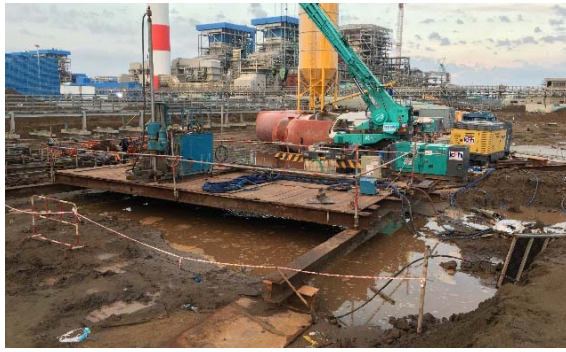
Figure 8. Jet grouting work in Duyen Hai 3 Thermal Power Plant
